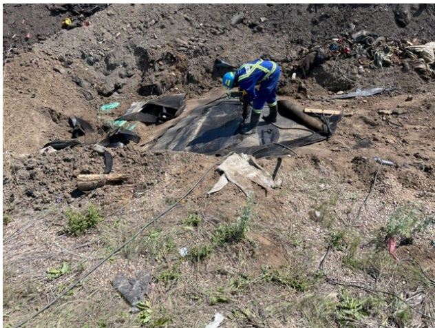
Repair in Progress
