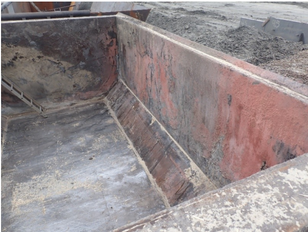
(Photo 3) Overview Of West Wall
