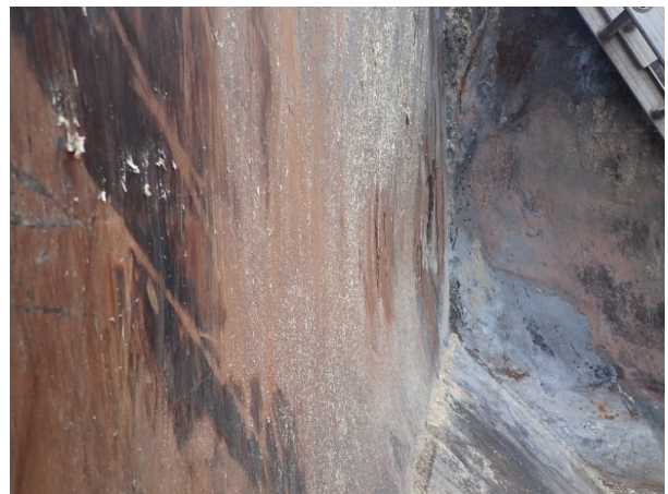
(Photo 6) General Shell Condition
